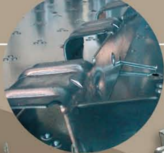
galvanized metal plank antiskid rustication and draining holes
